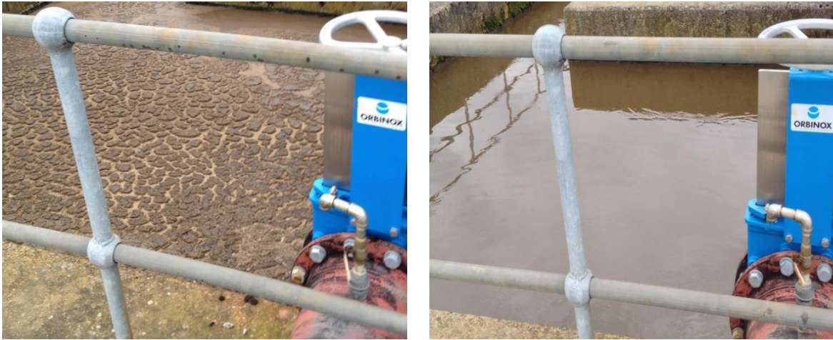
Figure 3: Performance of the ultrasound system on the anoxic zone 5 weeks after commissioning.
